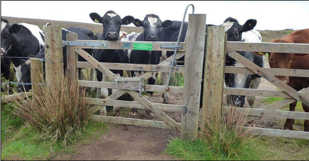
Carnyorth Common – new gates installed in 2008 across a public right of way to Tregeseal Stone Circle obstructed by a herd of cattle.
