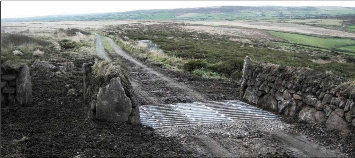
(08.C) December 2008: National Trust cattle grid later removed as being a breach of the Highways Act 1980
